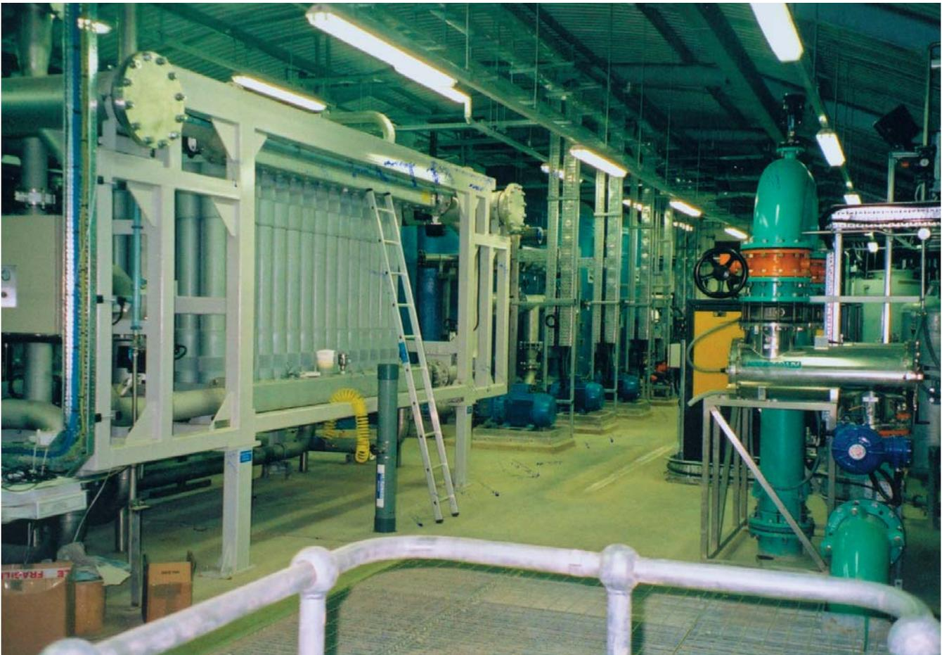
Membrane treatment skid (lhs) & UV treatment tubes (RH); module test equipment in foreground (courtesy Vivendi Water Partnership)
