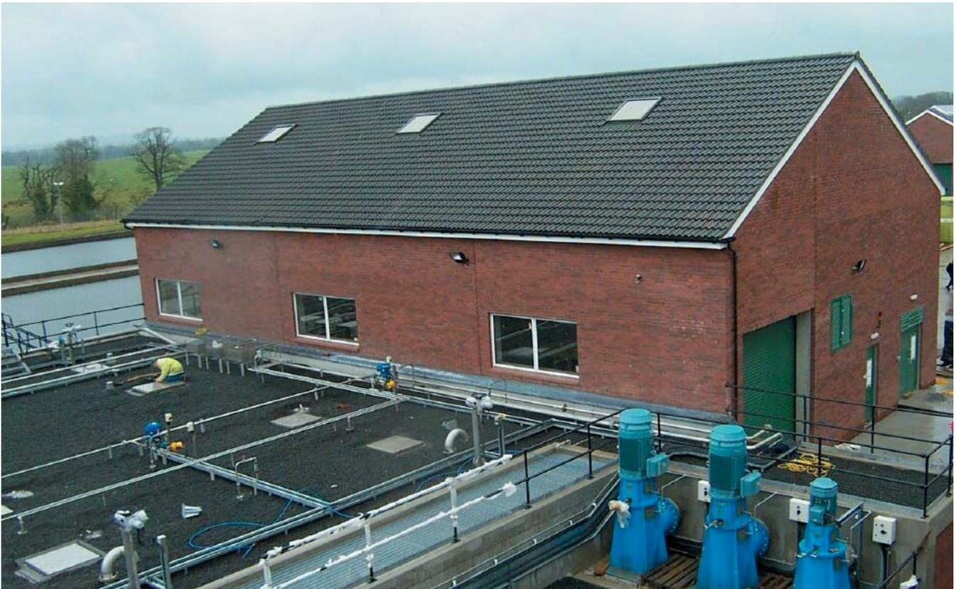
Rear view of plant from left to right: liquid oxygen compound, main plant building, 2nd stage contact tanks with first stage contact tanks to rear (courtesy Water Service)
