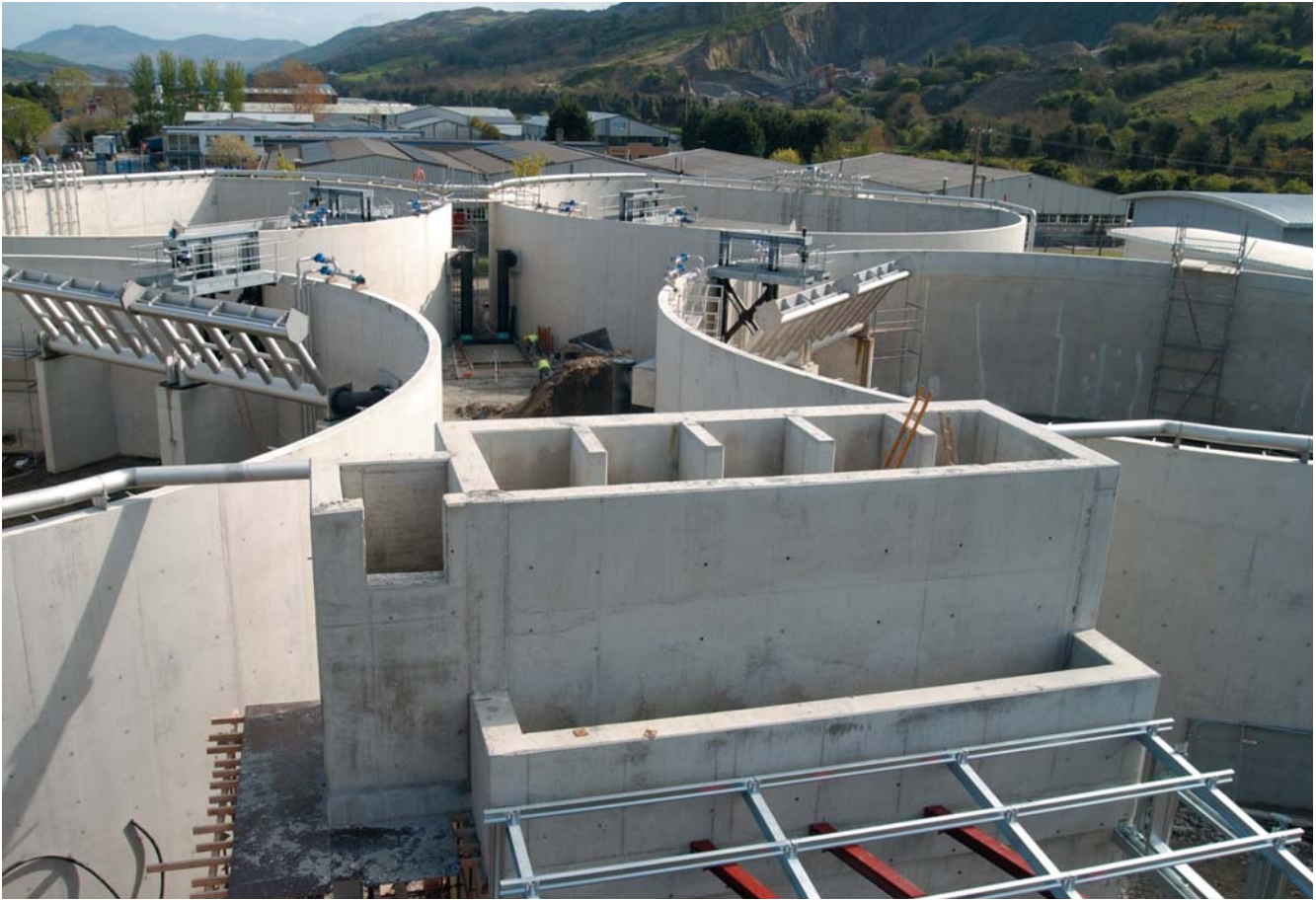
Newry WwTW under construction. (courtesy Ferguson McIlveen)
