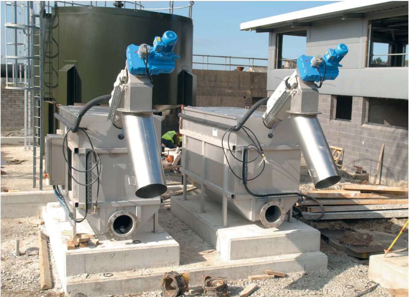
Newry WwTW under construction. (courtesy Ferguson McIlveen)
