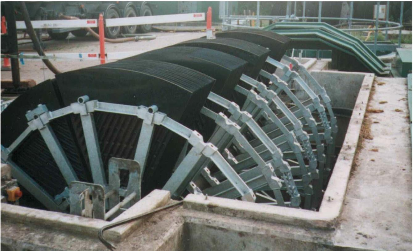
Copa rotor being assembled on site (courtesy Copa Ltd)
