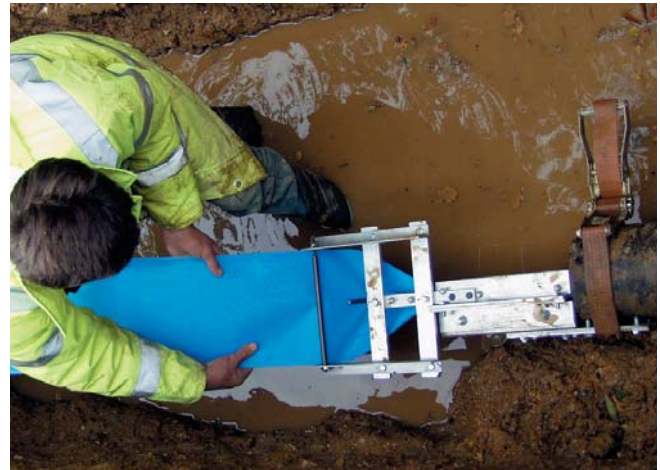
PE Liner prepared for insertion (courtesy Pipeway Ltd)
