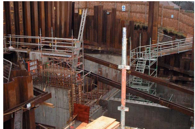
Pumping station under construction (courtesy Scottish Water)
