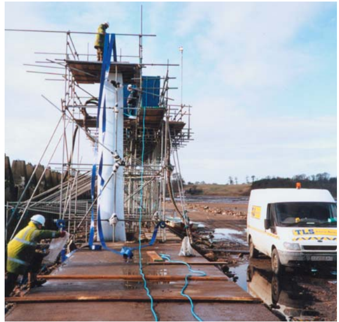
Construction work at Cramond (courtesy Scottish Water)
