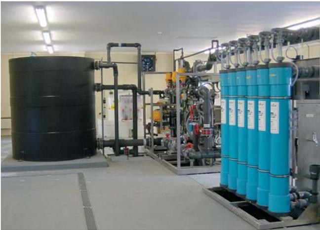
Ultrafiltration Pathogen Barrier (courtesy PCI Membrane Systems)
