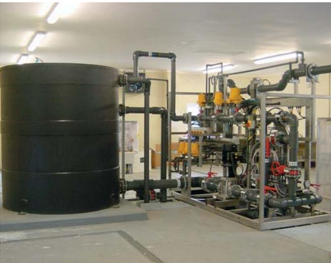
Membrane Cleaning (courtesy PCI Membrane Systems)
