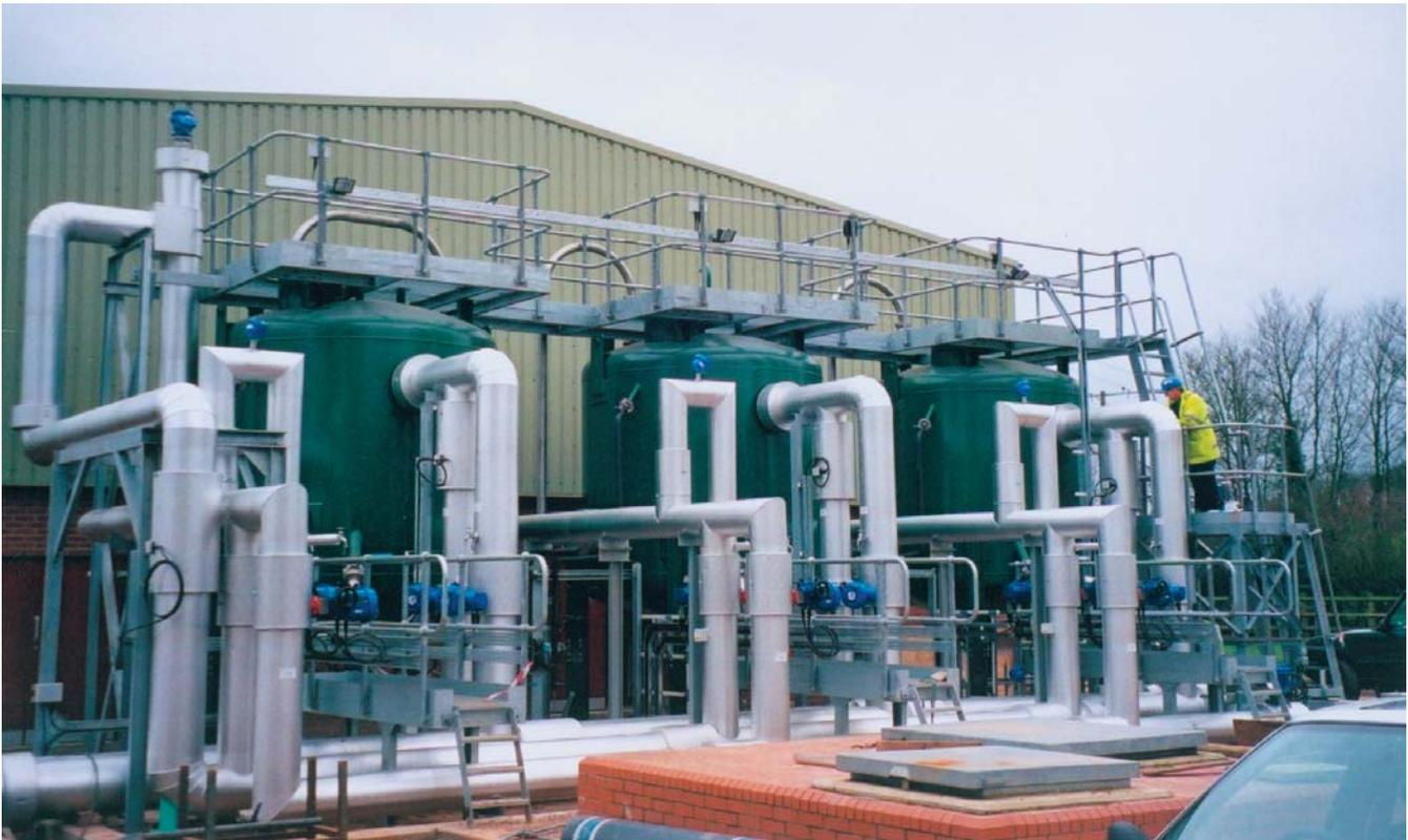
EWT adsorber vessels (courtesy Severn Trent Water Ltd)
