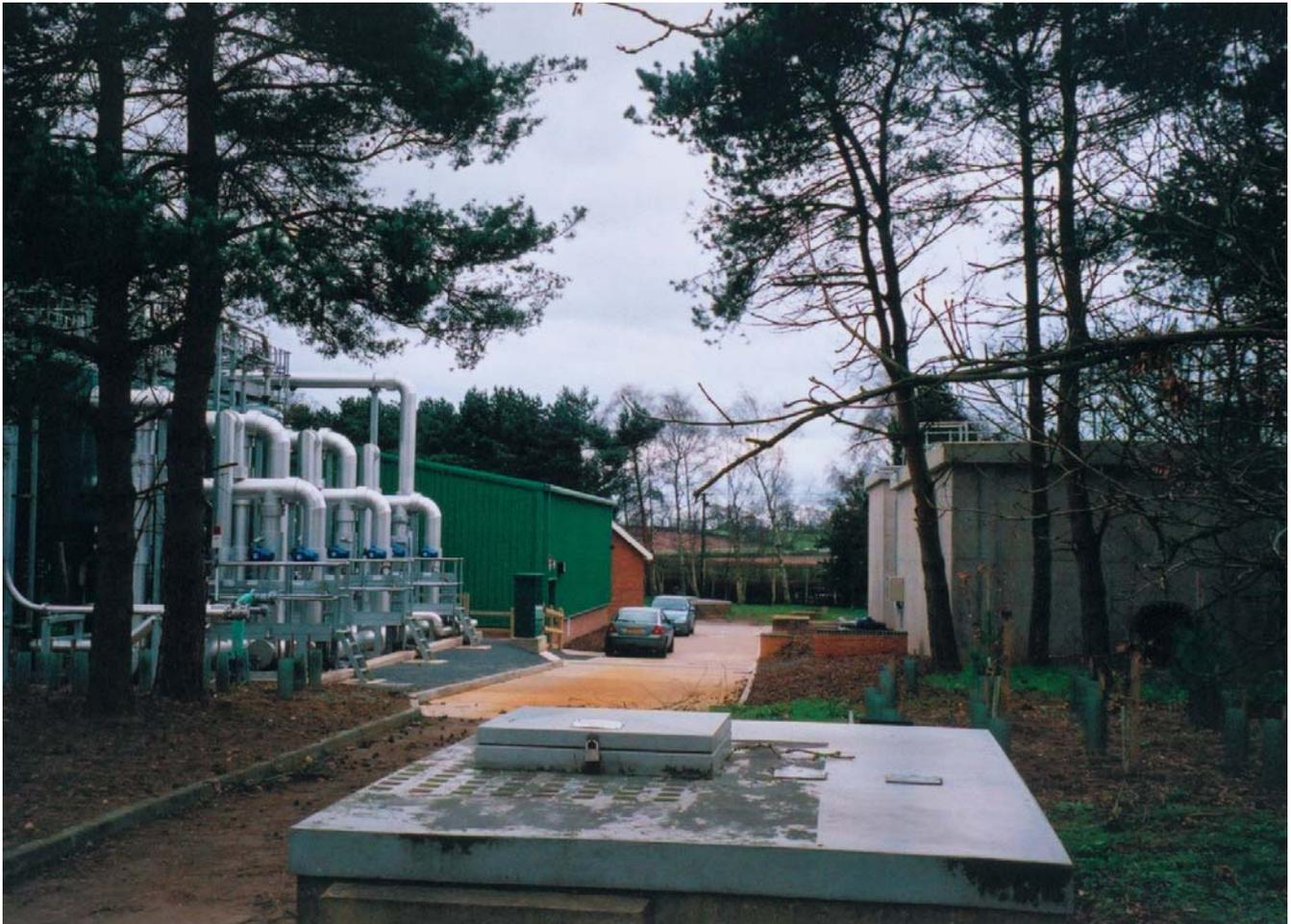
EWT plant showing adsorber vessels & reinforced concrete tanks (courtesy Severn Trent Water Ltd)
