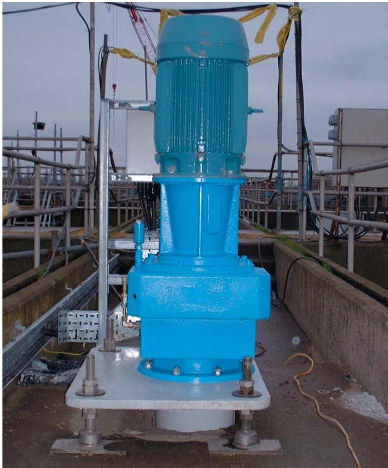
New vertical shaft aerator gear box (courtesy Thames Water Utilities Ltd)
