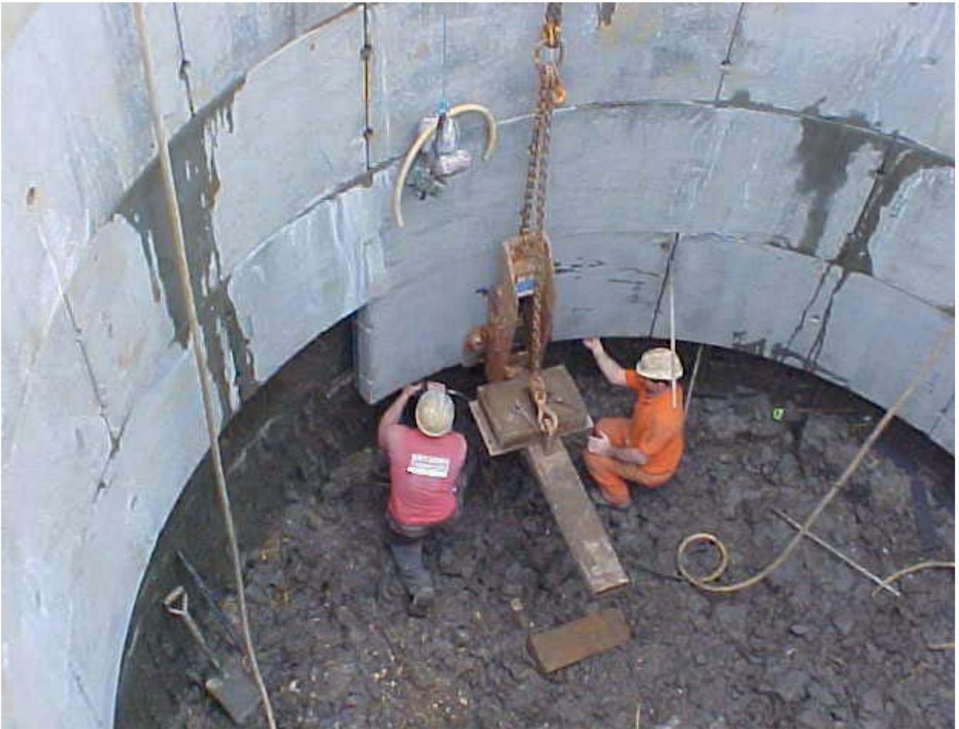
Segment being raised into position using Charcon's underbuilding frame ideal for use in very stiff weathered London Clay (courtesy Thames Water)
