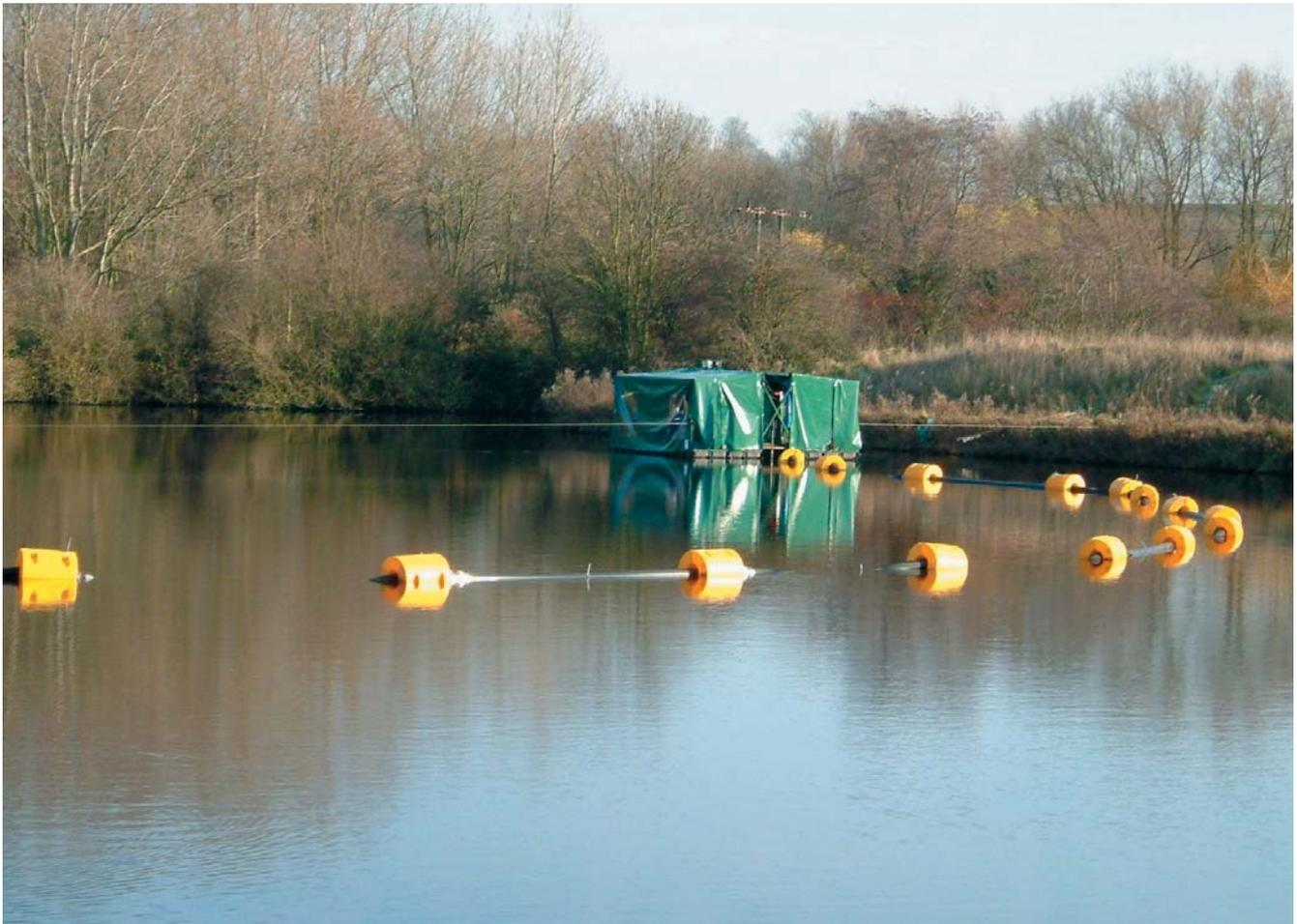
Dredger showing floating discharge pipeline & guide cable (courtesy Thames Water Utilities Ltd)
