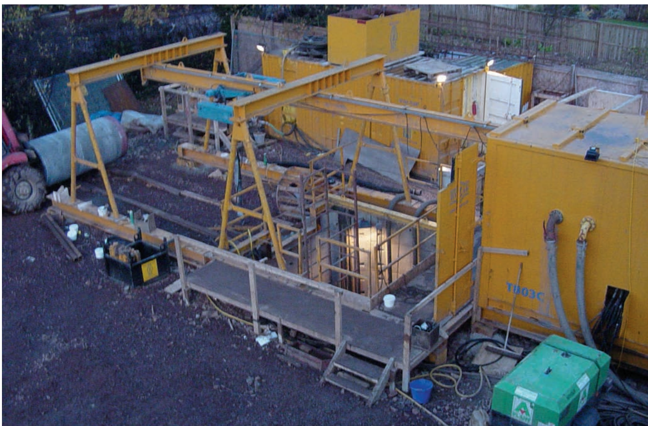
Tunnel set up shaft D (courtesy Hyder Consulting).
