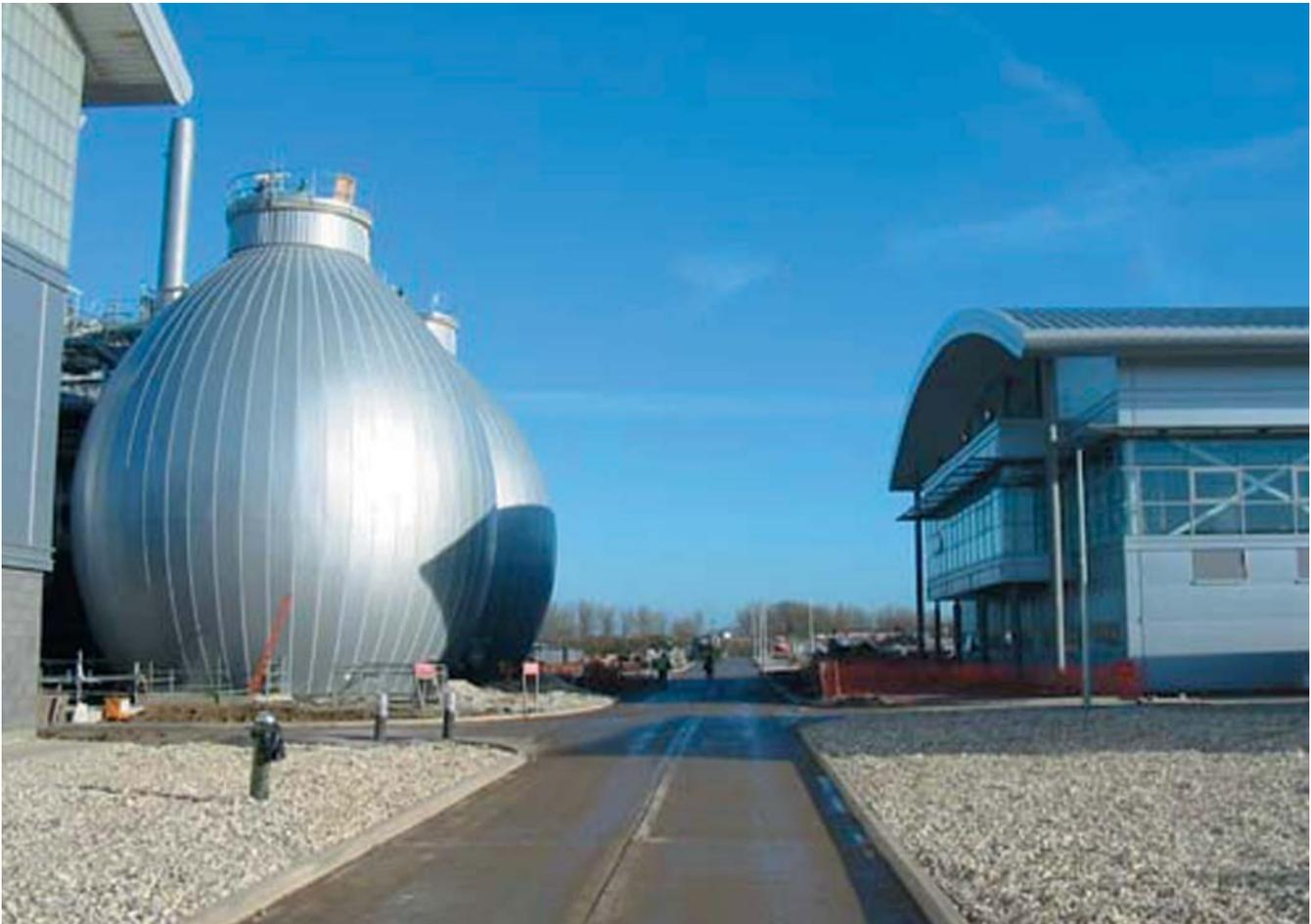
Reading STW: Site view of digesters with completed insulation and cladding
