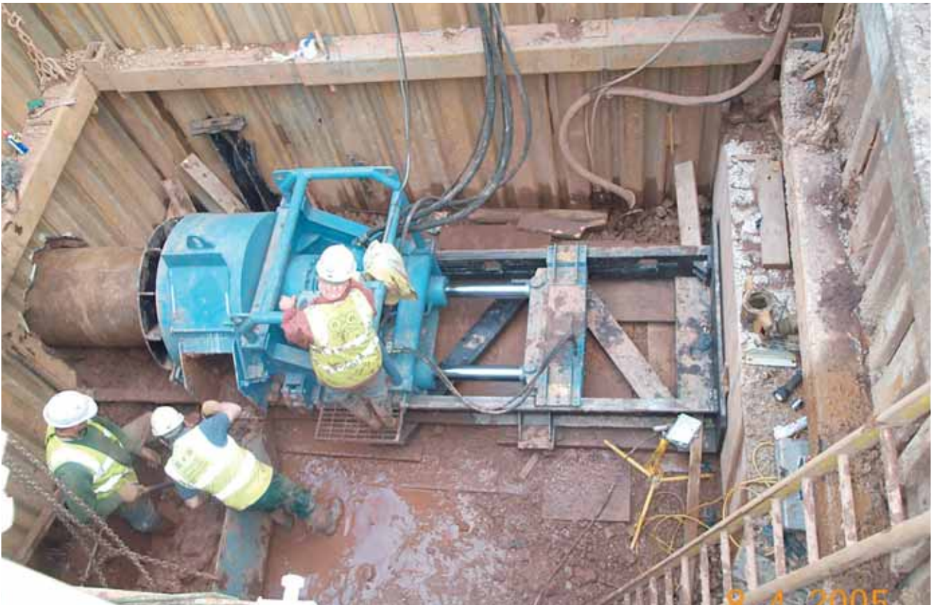
Huxley Green CSO under construction
