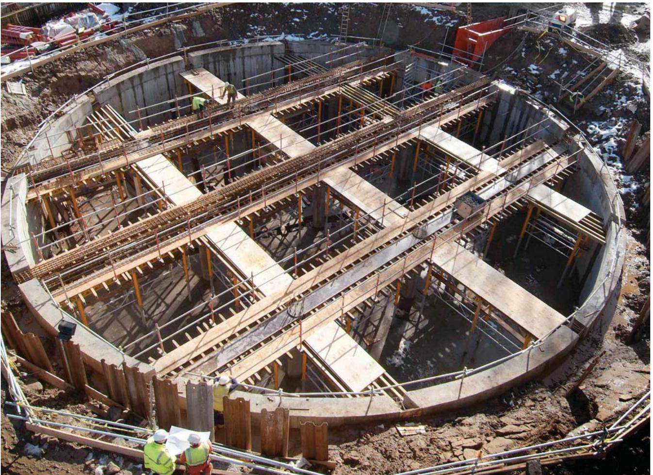
Moorside South, Fenham: 25m dia. storage tank 6m deep solves flooding problem
