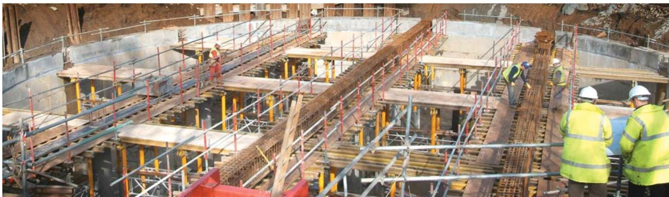
Storage tank 25m diameter x 6m deep giving storage area 1800m<sup>3</sup> to solve flooding problem
