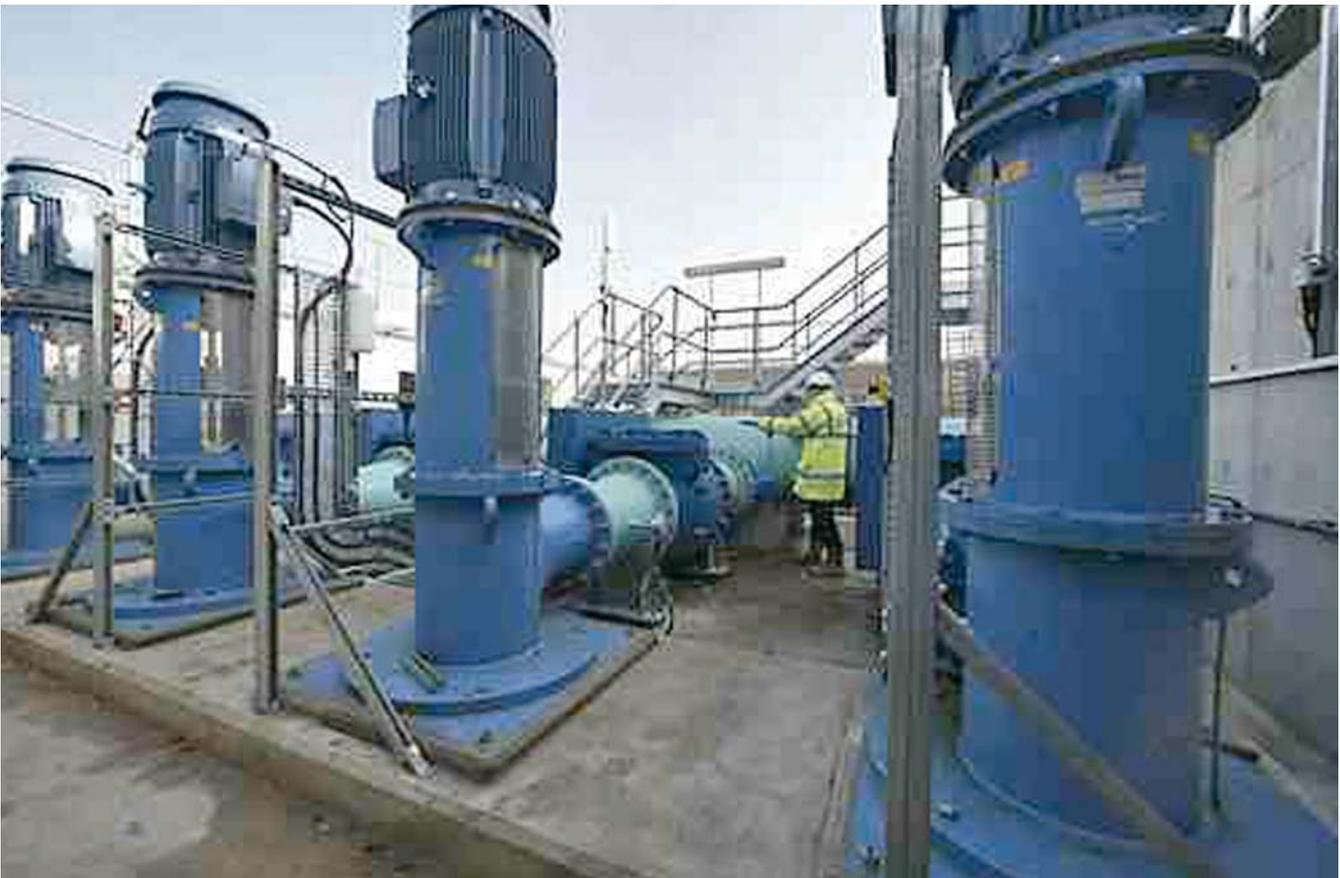
Prescot WTW: New filtered water PS with new pumps, pipework, valves & access steelwork
