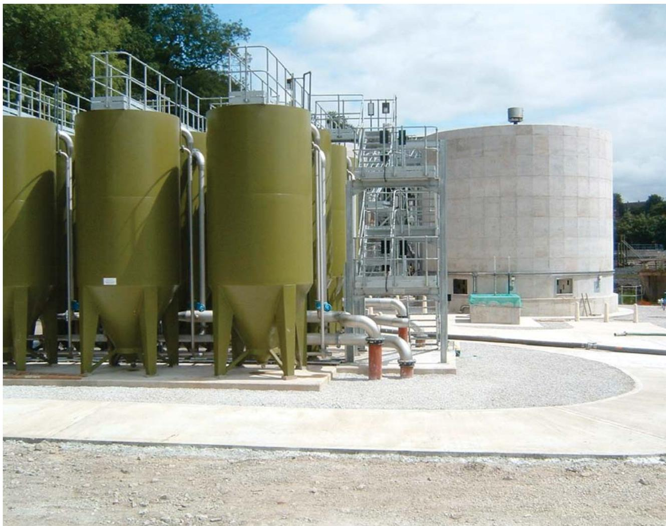
Wilmslow WwTW: Continuous Operating Upward Flow Filters (COUF's) and 10m diameter Nitrifying Trickling Filter
