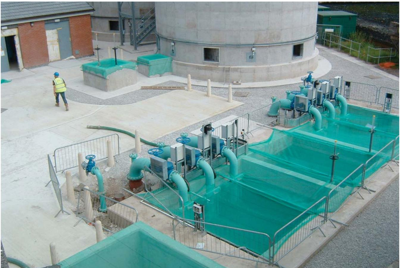
Wilmslow WwTW: Feed pumping station with above ground valve arrangement
