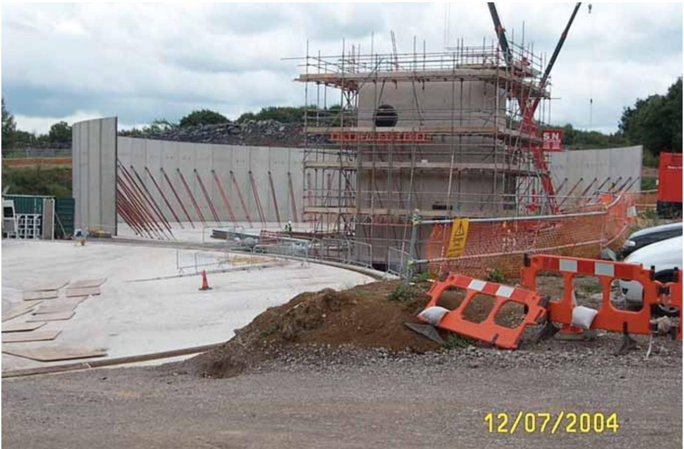
Construction of 45m diameter storage tanks at Salford STW
