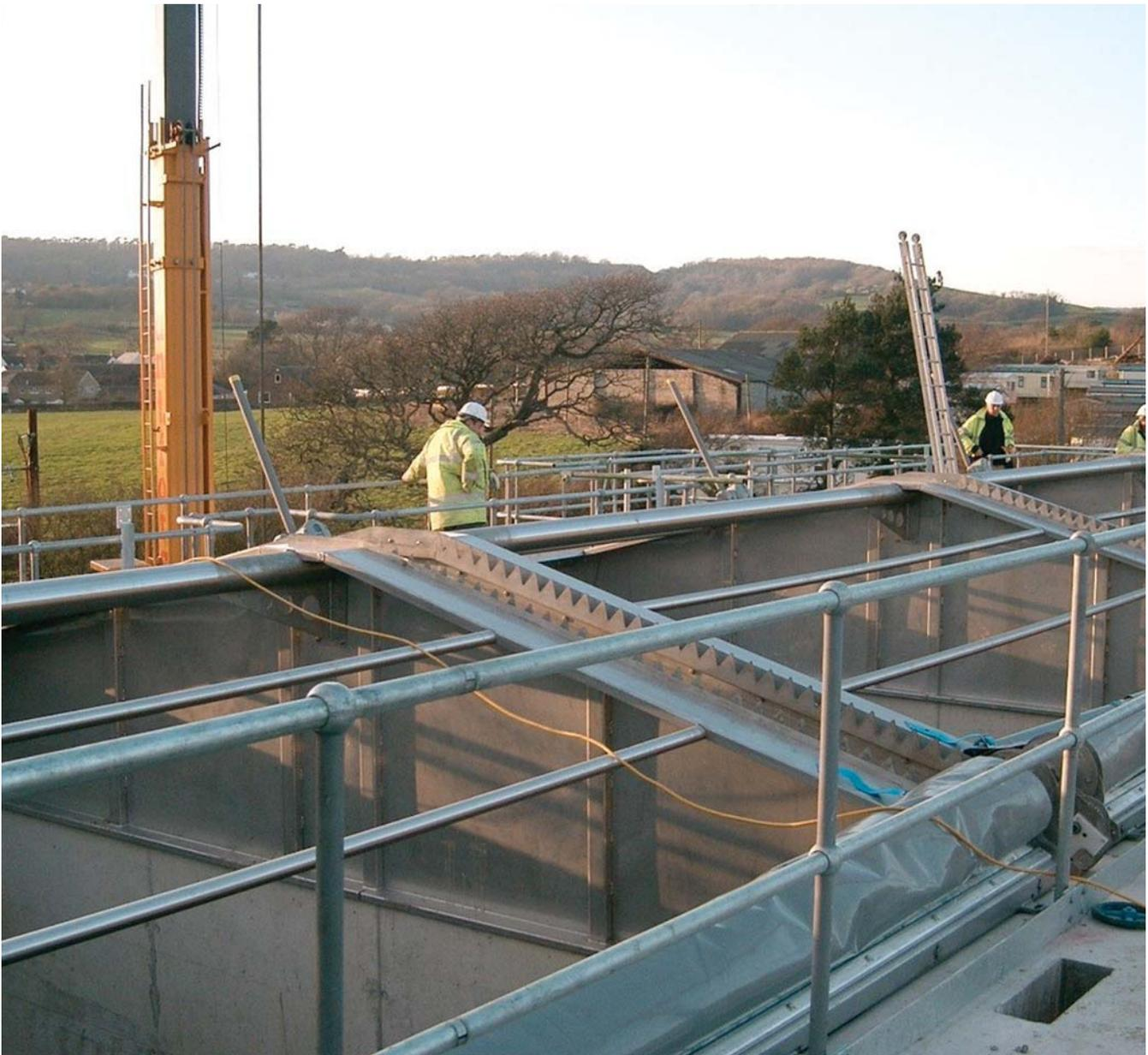
Charmouth STW: Rollback covers fitted to SBR tanks
