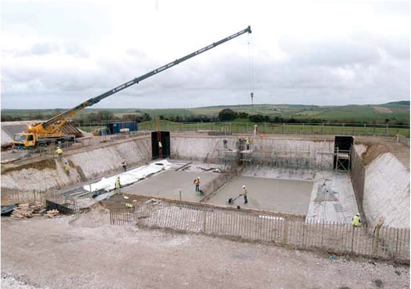
Dorchester: New service reservoir under construction
