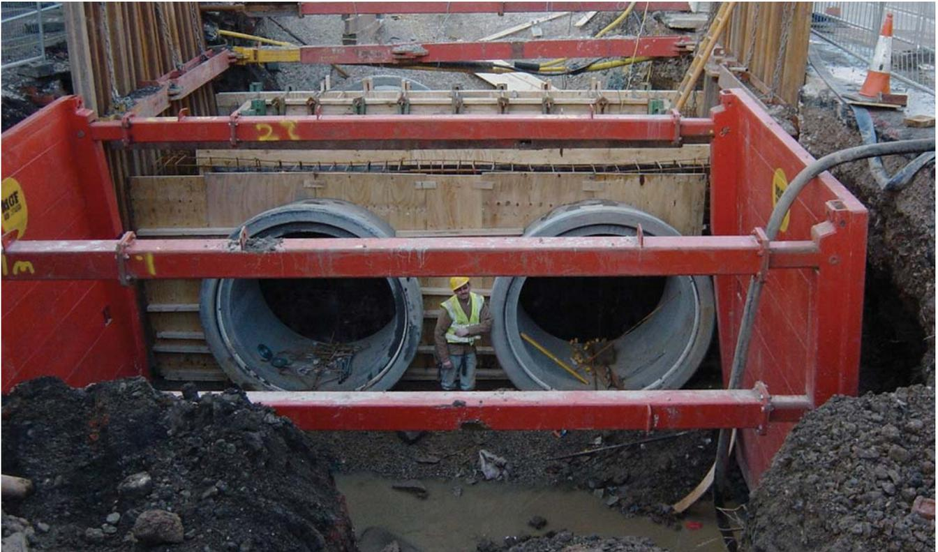
Totley Brook Road: Twin 1800mm pipes being installed in urban area
