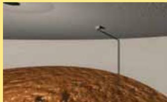
STEM Drive® a range of patented fluidic mixers for sludge holding tanks, detention tanks, storm tanks and digesters. Controls odours and eliminates stratification within sludge tanks. No moving parts within the tank. External air or gas power source. Live tank installation an option.
