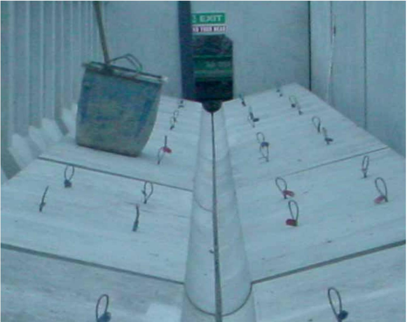
Merthyr Dyfan CSO: Placement of pre-cast batters, forming benching of one of side channels.- laser measured for accuracy
