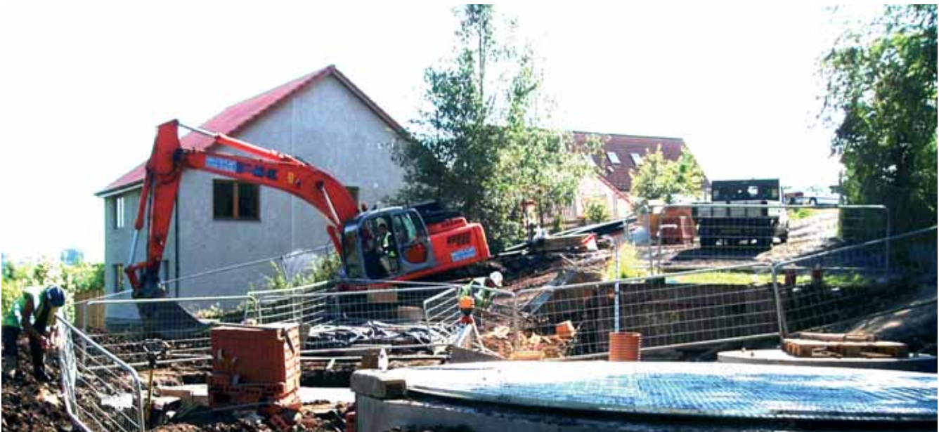
Pitscottie WwTW: Underground SAF being constructed
