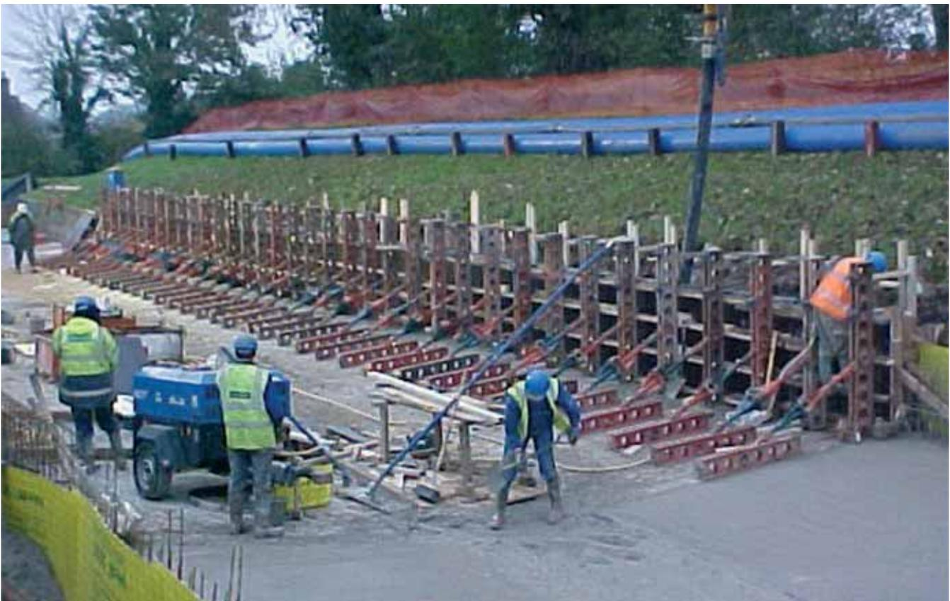
New River: Construction of new walls - overpumping pipes on embankment
