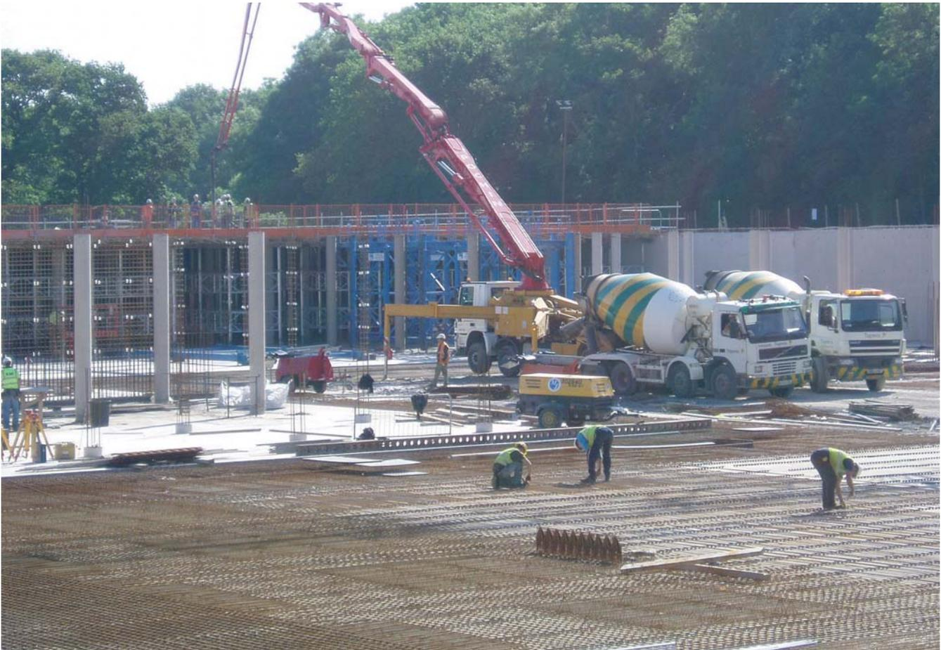
Northern Strategic Support Scheme - reservoir under construction showing column casting rig
