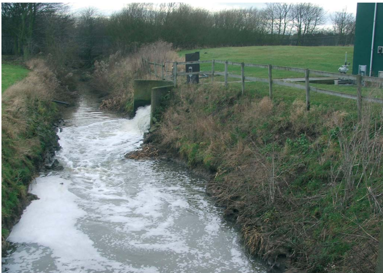
Existing discharge to Cowbridge Beck from Billingham STW
