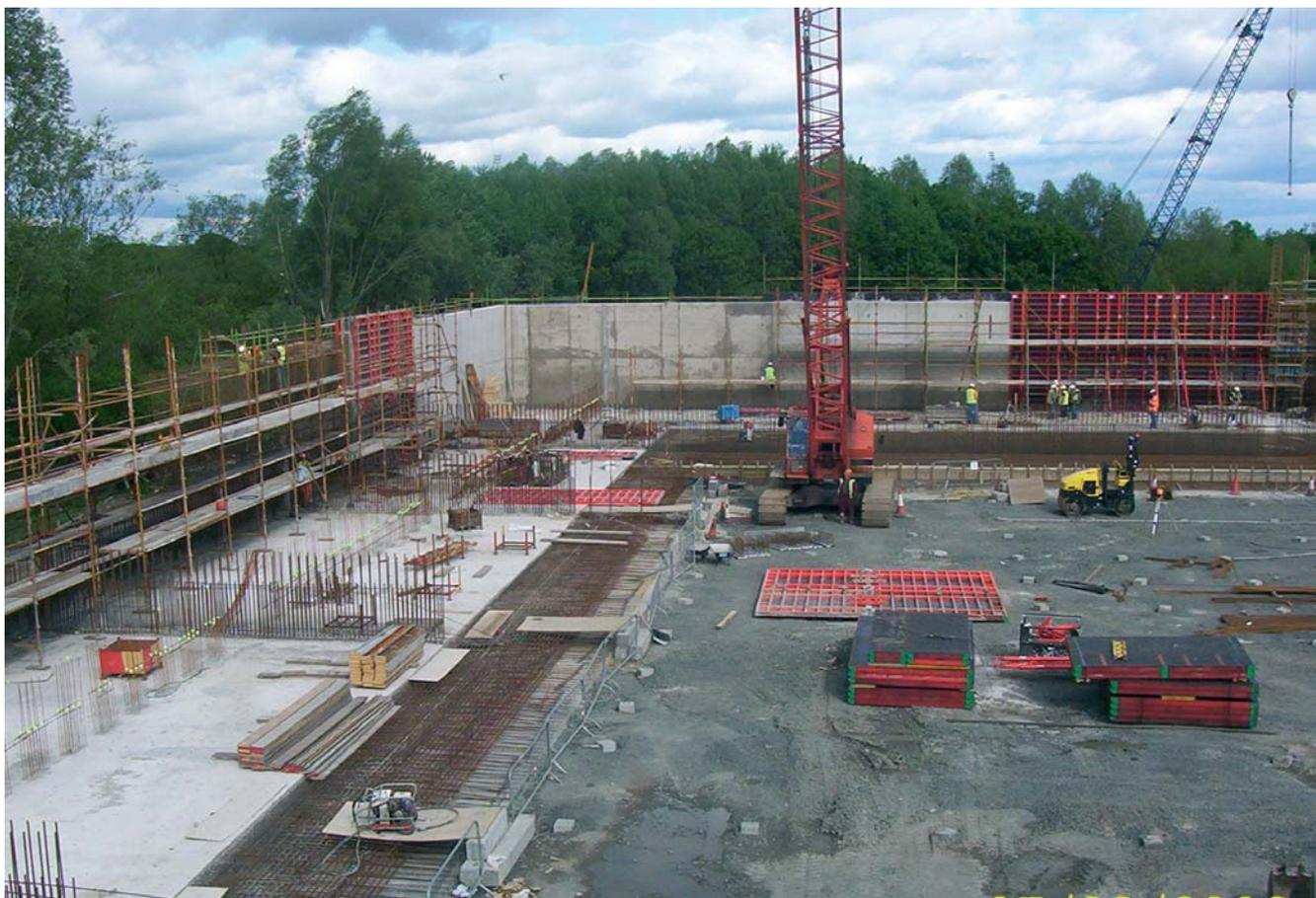
Phased construction progress of the SBR structure to maintain access for concrete pours
