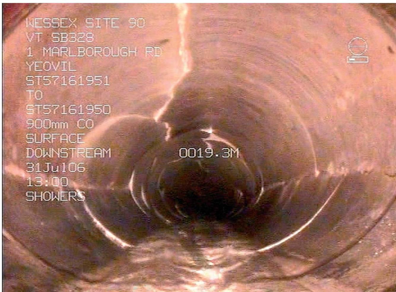
Yeovil: View inside deteriorated storm water sewer showing the fracture failures
