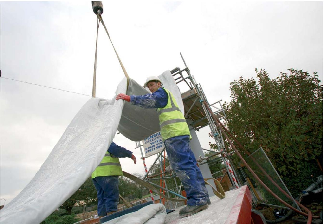
Feeding the liner into the host pipeline during the installation phase of lining
