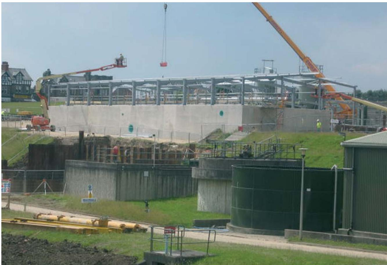
Erection of steelwork frame to newly constructed rapid gravity filter substructure
