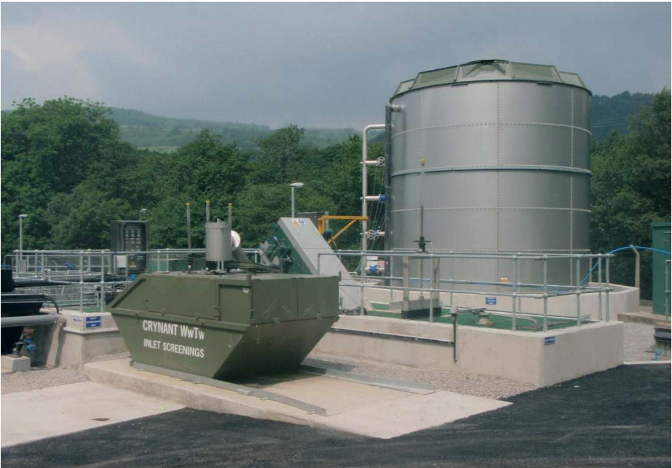
Circular storm tank modified for re-use as Primary Settlement Tank photo courtesy Dwr Cymru Welsh Water
