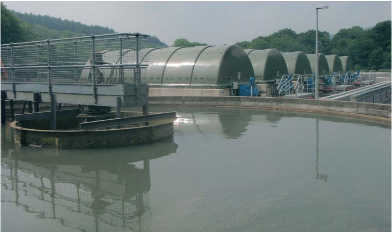
Storm tank as Primary Settlement tank & 6 RBC's to achieve carbonaceous oxidation & nitrification
