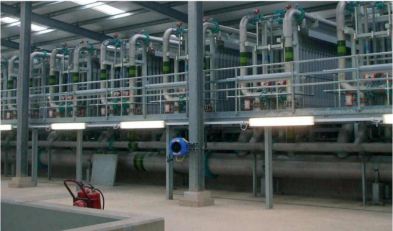
Photo inside membrane plant building showing arrangement of membrane units & mezzanine access platform
