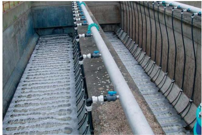
Pattern test on high efficiency diffusers during Commissioning tests Courtesy of the @one Alliance
