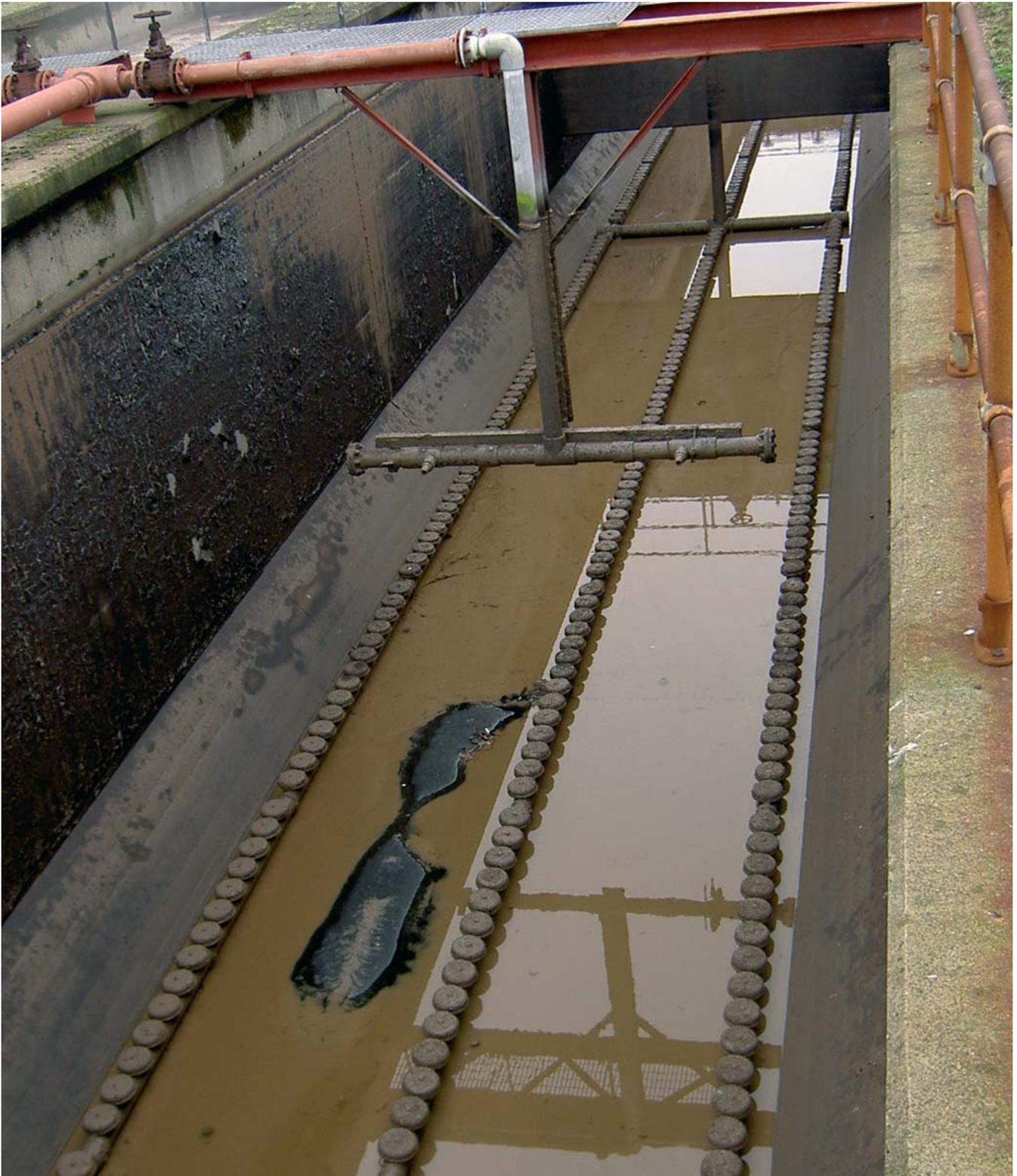
*Old works' disc diffusers in drained wide lane before replacement*
