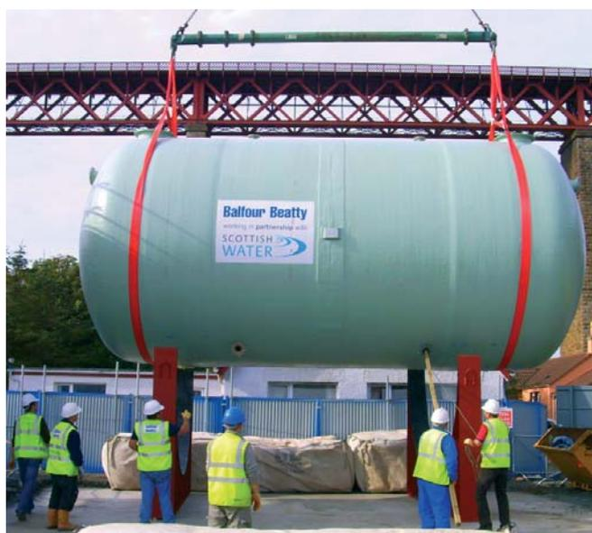
Four 100,000-litre GRP septic tanks were installed as part of the project
