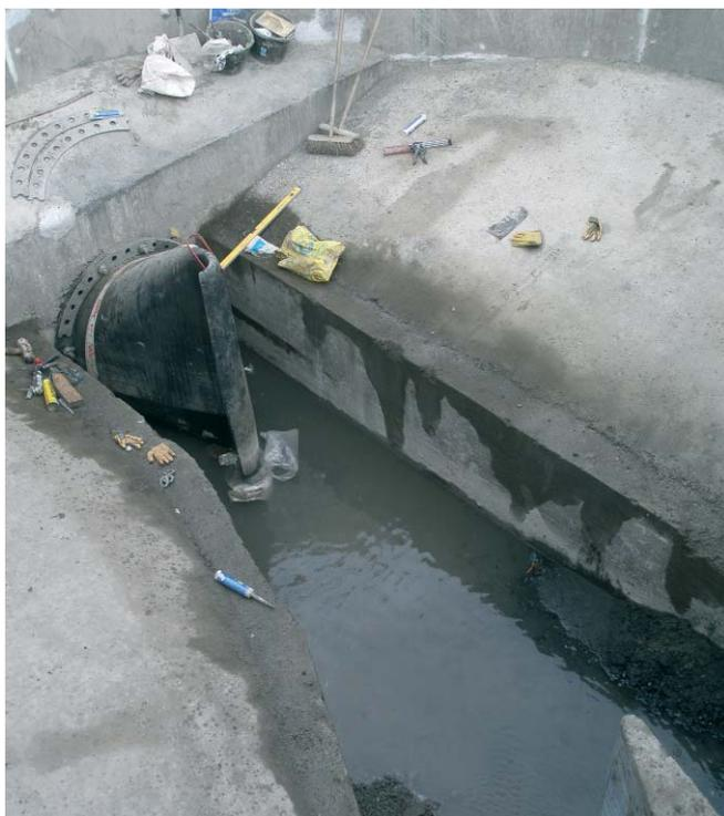
The same Overflow Connection Chamber nearing completion, showing the "Tideflex" non return valve on the 1.05m diameter inlet pipe.
