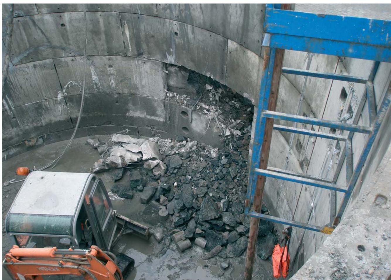
*Mini excavator with breaker breaking hole in a 7.5m diameter, 7.0m deep Overflow Connection Chamber shaft for a 1.05m diameter inlet pipe.*
