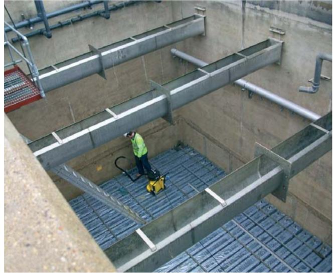
Installation of Leopold Floor in GAC Contactors
