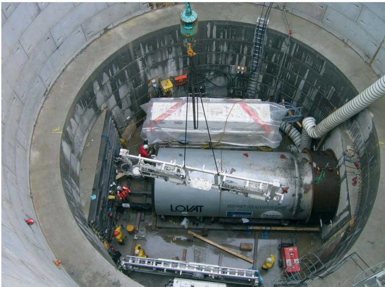
Photograph looking into the shaft down on to TBM
