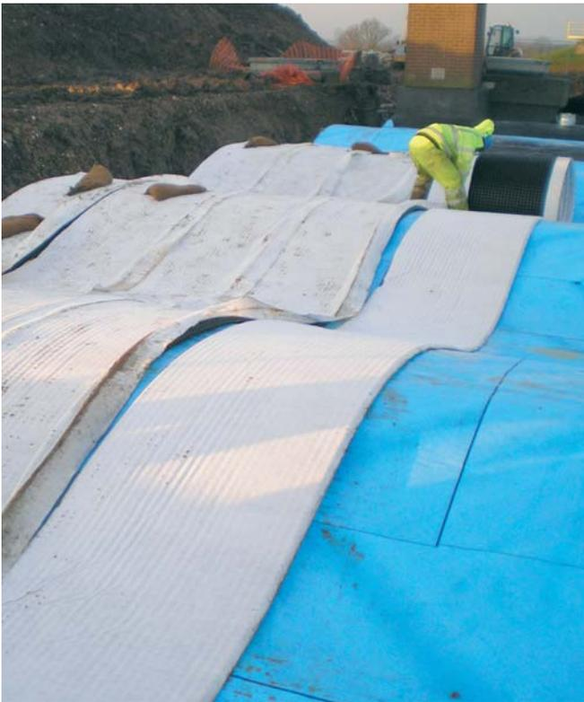
Installing geocomposite drainage layer over new waterproof membrane
