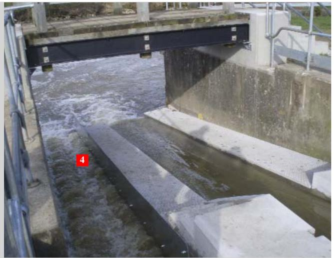
3 Fish Pass (note baffles) 4 Fish Pass baffles controlling flow
