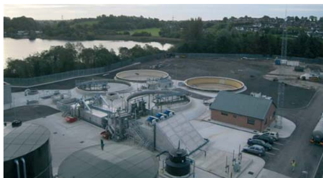
Aerial photograph of Enniskillen WwTW
