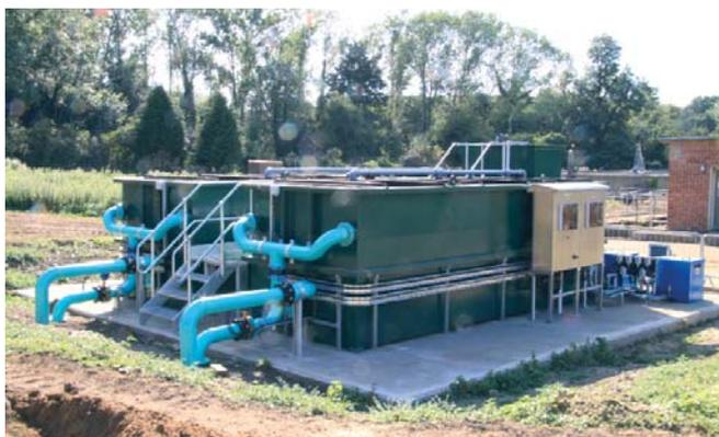
HSAF Solids Filter built for Anglian Water as part of a P removal project
