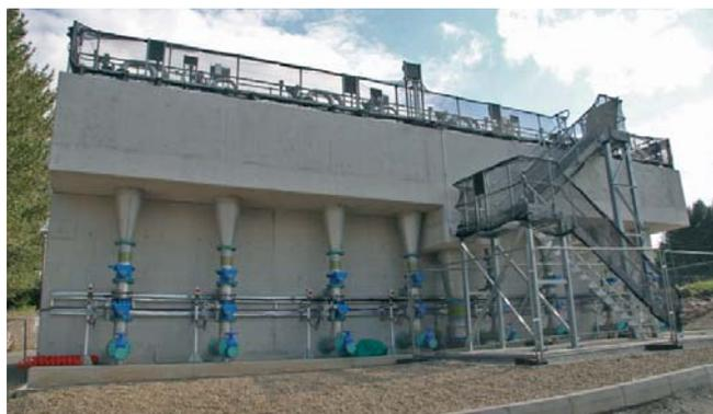
Large Scale HSAF delivering consent compliance at 1 mg ammonia/l on a 95%ile basis, whilst using only one third of the power of alternative SAF technology, built for United Utilities
