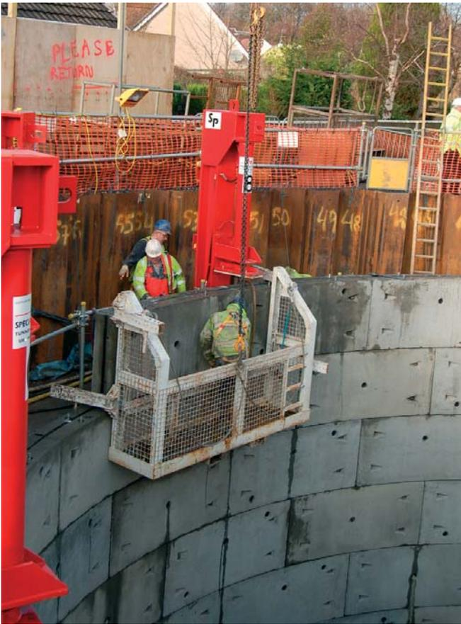
Jacking in Operation within the clearly constrained site Courtesy of Scottish Water Solutions
